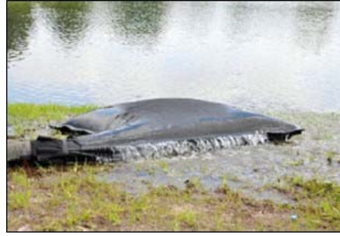
Plate 4-4 Silt bag under inspection
