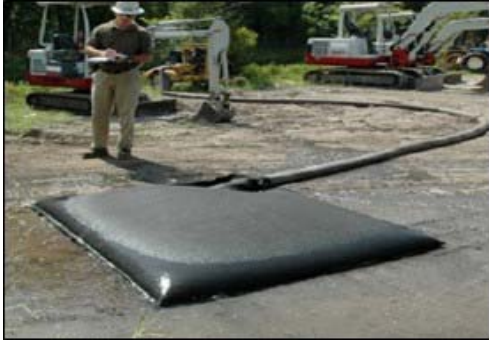
Plate 4-3 Silt Bag with water being pumped through
