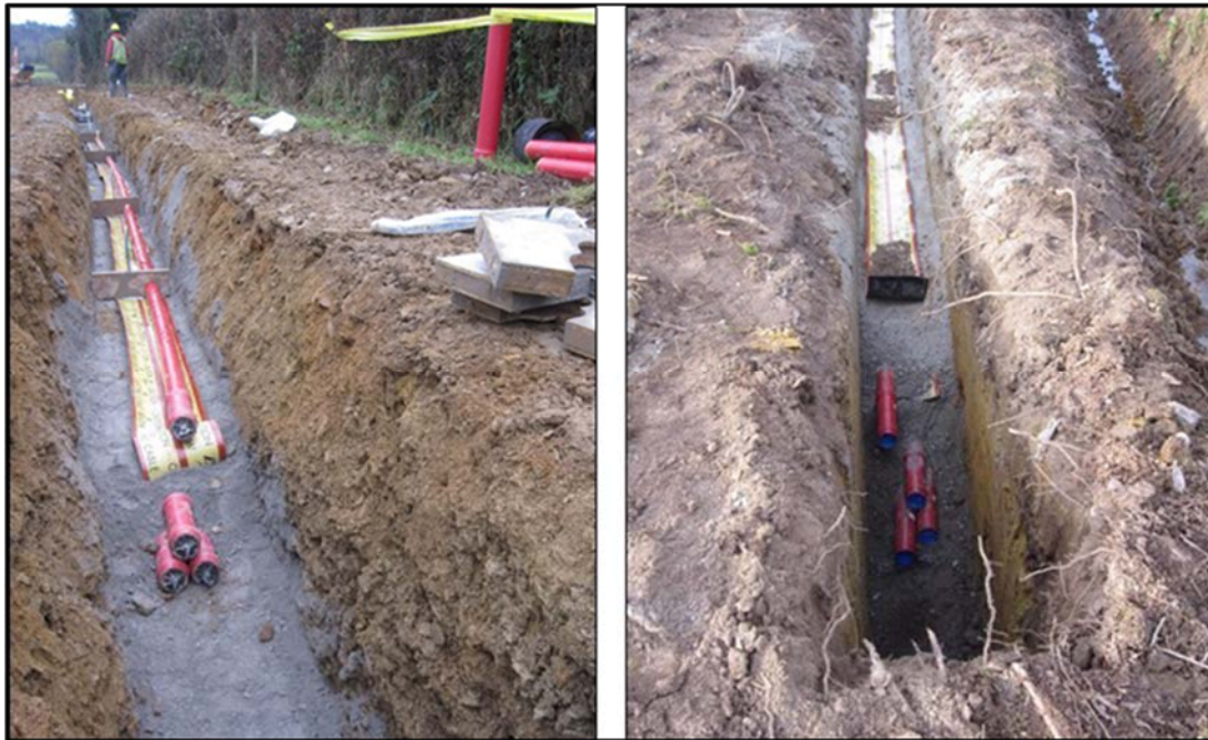
Plate 4-5 Typical Cable Trench View
